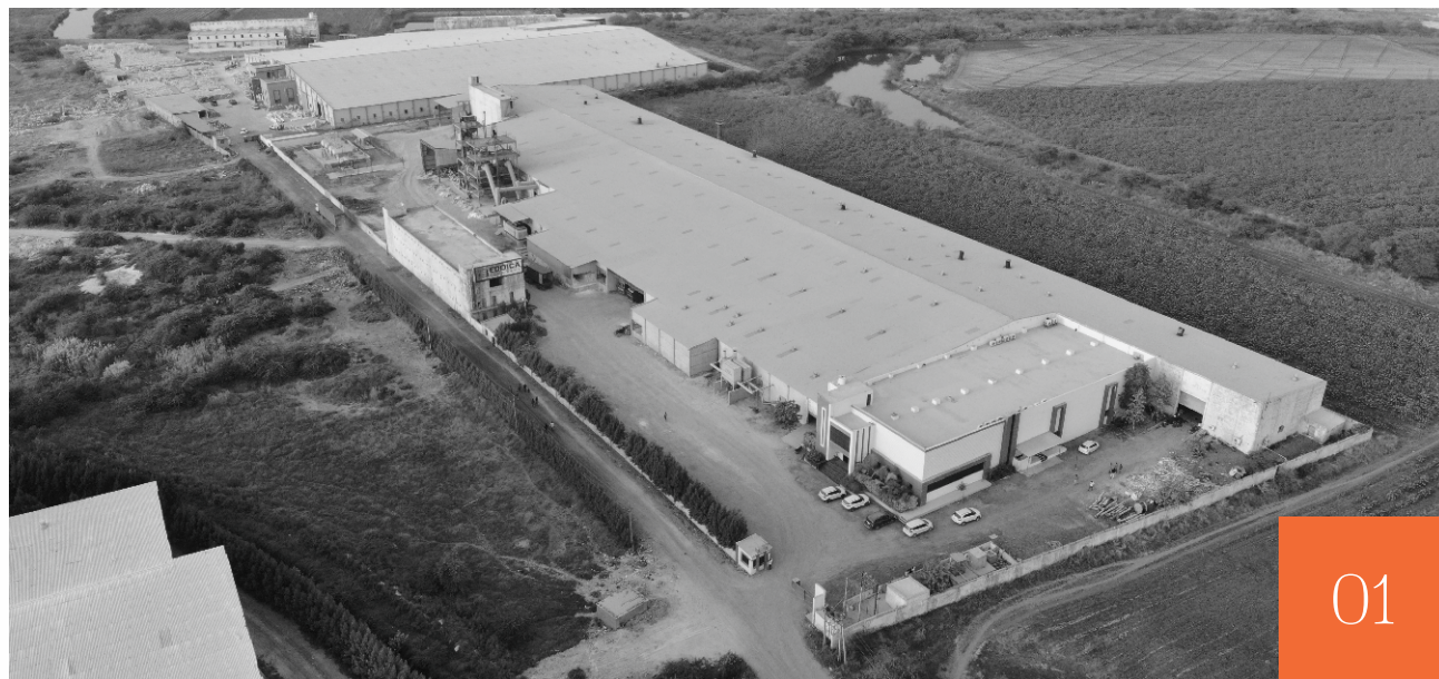
EXCLUSIVE TILES FACTORY
